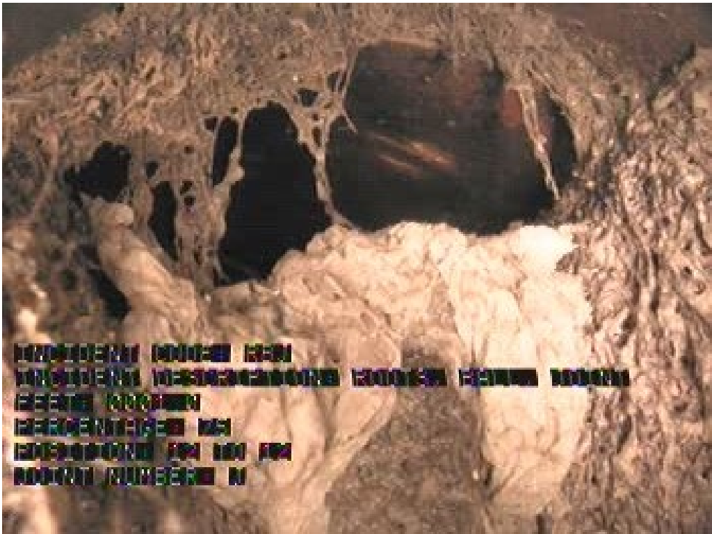
Root ball just upstream of manhole 2-77. WIB cause possibly root ball.
